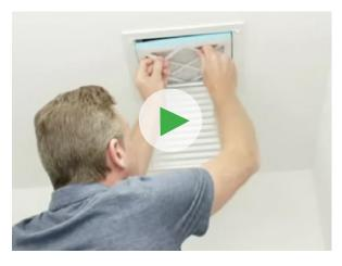
**The Lesson:** When installing air filters in HVAC systems in the dental office setting, choose the highest possible MERV level that the HVAC equipment can accommodate. If the HVAC units cannot accommodate the resistance of filters with appropriate ratings, MERV 13 or above, the ASHRAE, recommends upgrading HVAC systems and/or achieving equivalent airflow by adding separate filters and air cleaners.
